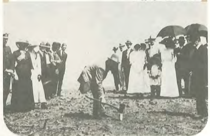
Pegging the site, 1913
