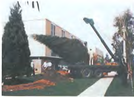
Instant landscape—a 7m tree is lifted into place
